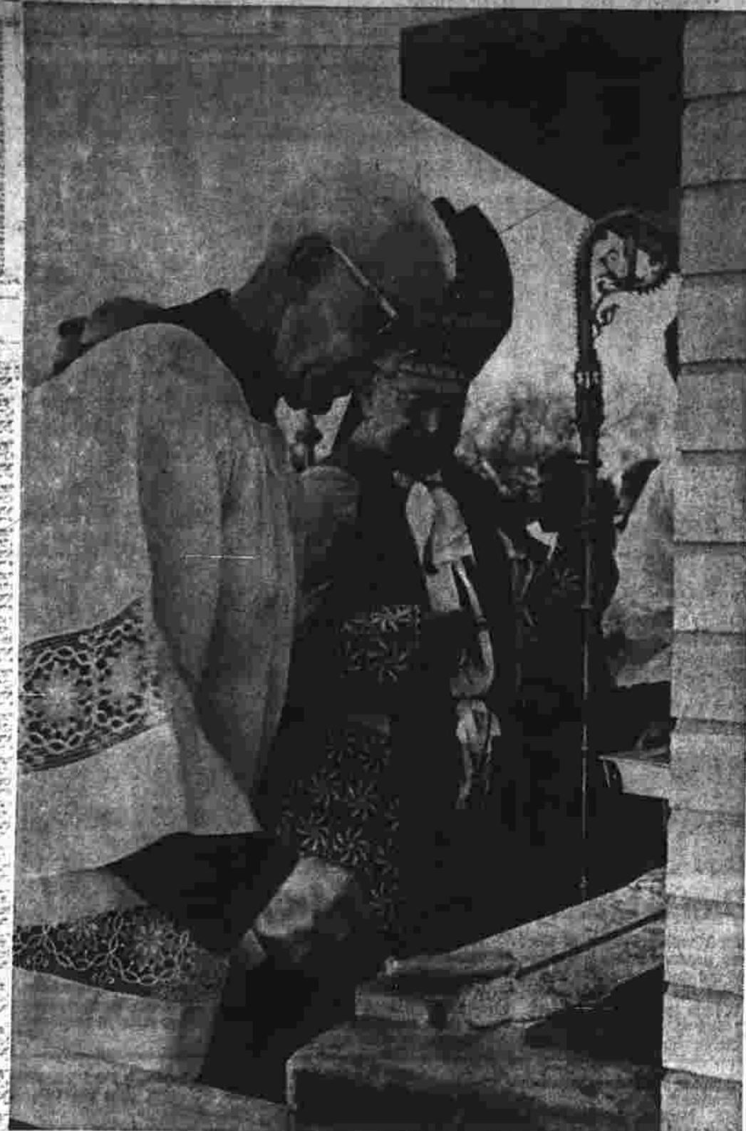
Wielding the same silver trowel that had been donated by Cheney Bros. for the cornerstone-laying of the present church edifice in 1896, Father John Delaney, pastor of St. Bridget, spreads mortar on the cornerstone of the parish's new school. The Most Rev. Henry J. O'Brien, Archbishop of Hartford, who applied the first touch of mortar, then blessed the stone. (Herald photo by O'Hara.)
